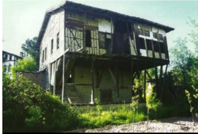
Figure 5. A Mansion Constructed Wooden Frame with Adobe Filling(BURKUT, K. 1996)
